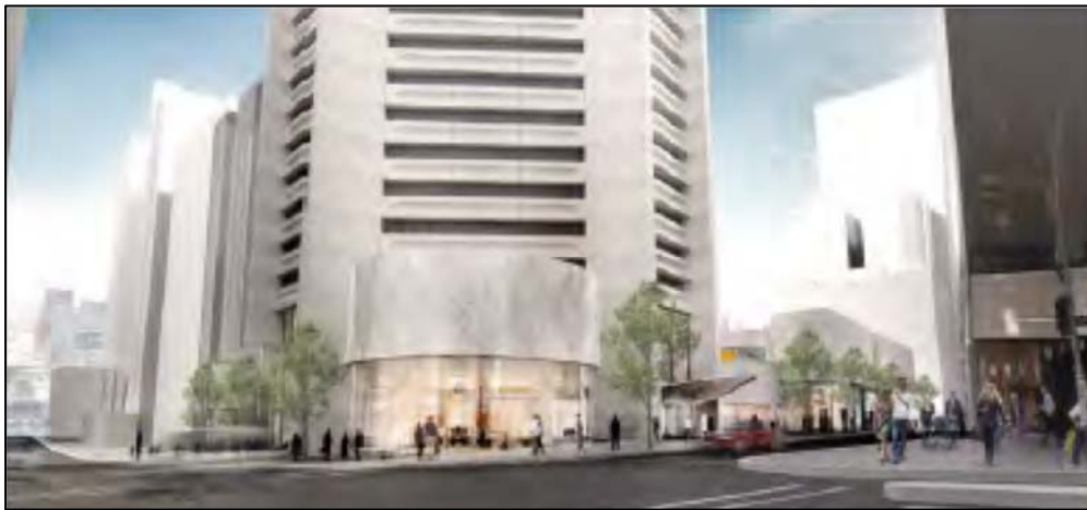
Figure 20: The scheme presented to the DAP sub-committee, as viewed from the corner of King and Castlereagh Streets
