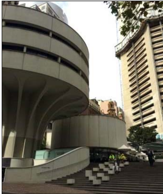
Figure 3: View of the CTA club and existing plaza level retail tenancies (Level 7) as viewed from Martin Place
