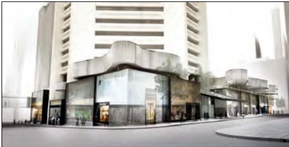
Figure 18: The original design concept presented at pre-lodgement stage, as viewed from the corner of King and Castlereagh Streets
