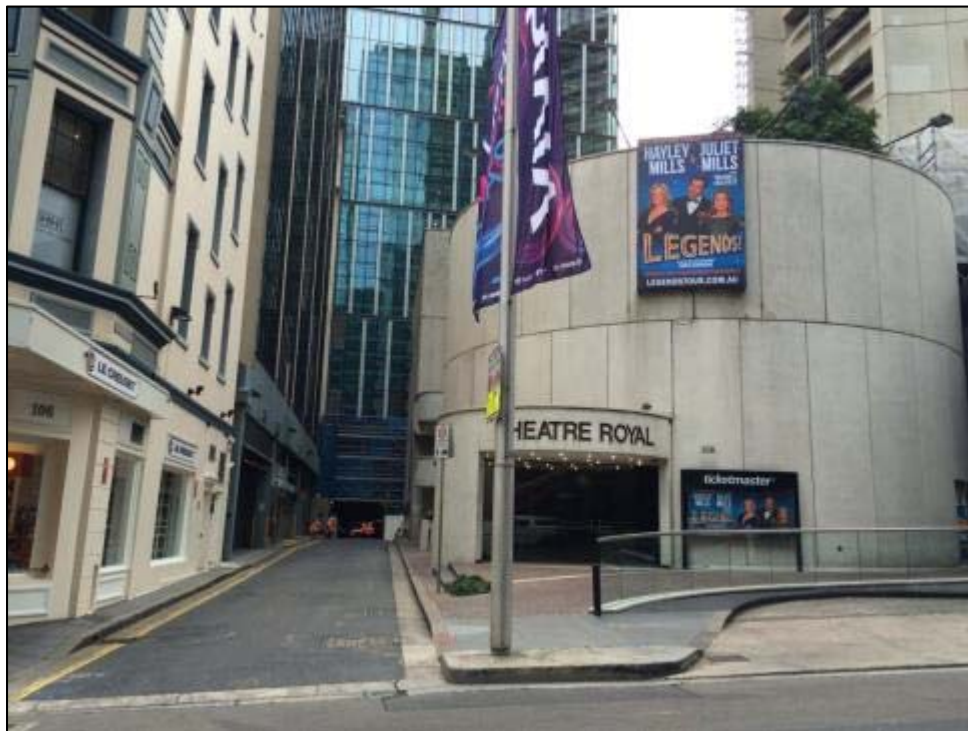
Figure 6: View of Lees Court, entry to the 'Theatre Royal' and vehicular entry to the site as viewed from King Street
